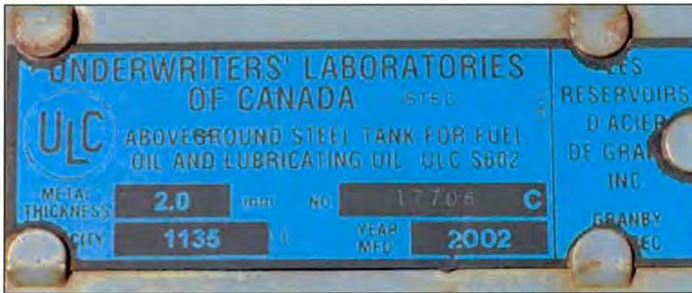
4.1a ULC certification plate: standard, single-wall, steel aboveground heating oil tank
