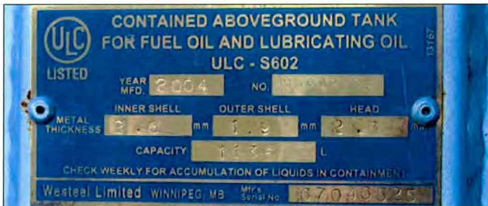
4.1b ULC certification plate: standard, double-wall, steel aboveground heating oil tank
