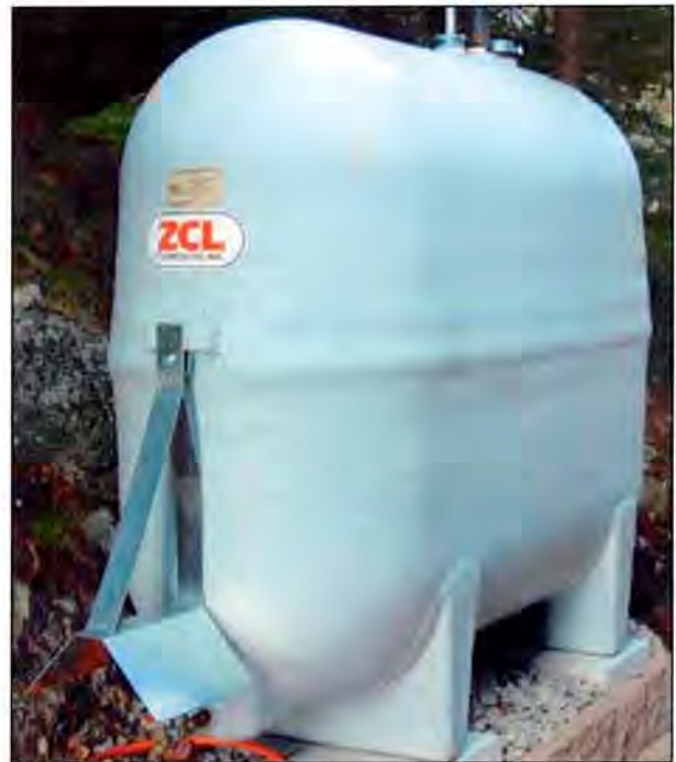
5.4 Fibreglass, 1,135 litre (250 gallon) single-wall heating oil tank. Note the protective shield over the fuel outlet valve. (Photo courtesy of ZCL Composites, Edmonton, AB.)
