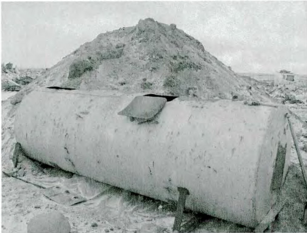
Photos 9 and 10 – Soils excavated and deposited at the community landfill site
