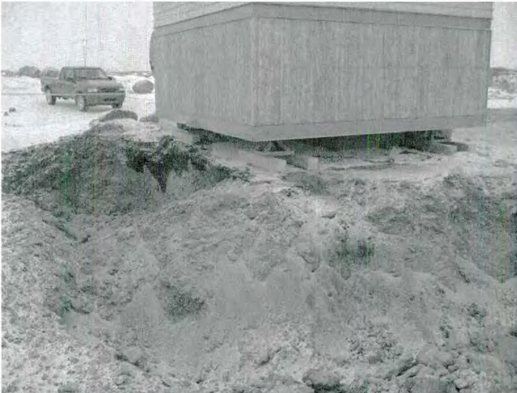
Photos 7 and 8 – Excavation work prior to Stabilis arrival on site
