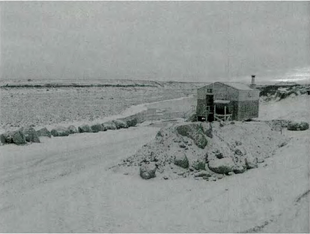
Photos 1 and 2 – North view of Tasiujaq pumping station and Disinfection plant
